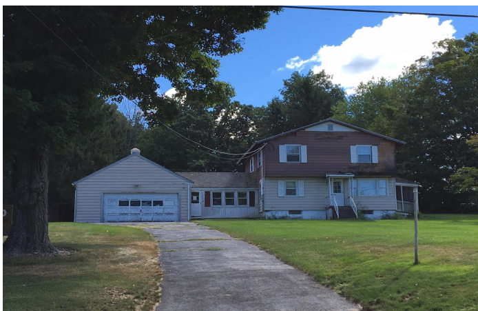
Out building +/- 2,000 S/F office/ house structure
